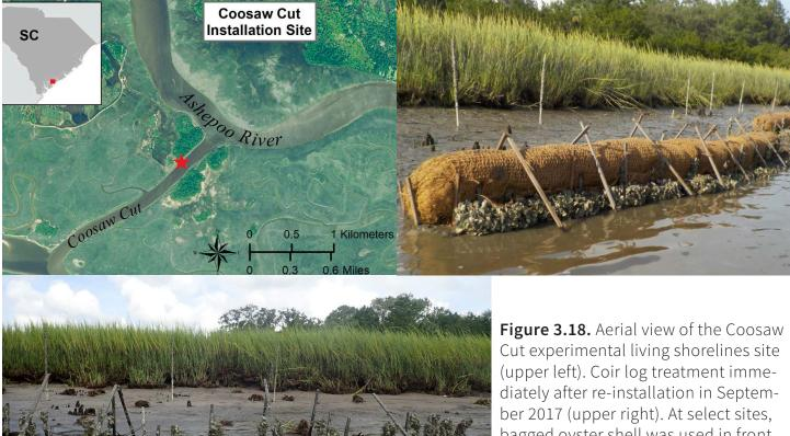
ber 2017 (upper right). At select sites, bagged oyster shell was used in front of the coir logs to prevent undercutting of the log (upper right). Missing coir logs with remaining oyster shell bags in September 2018 (lower left).
