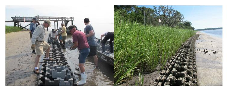
**Figure 3.21.** Oyster castle reef on Lucy Point Creek, near Beaufort, SC, shown during construction (left) and Coosaw River, near Beaufort, SC, shown 2 years after construction (right).
