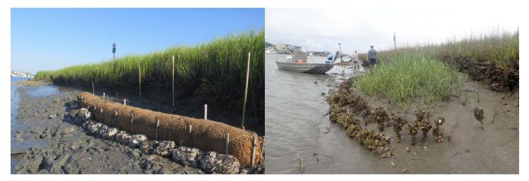
**Figure 5.2.** Single-row coir log treatment with a single row of shell bags, installed in July 2016 along Big Bay Creek (left). This treatment was planted with smooth cordgrass in April 2018 and photographed in May 2019 (right)
