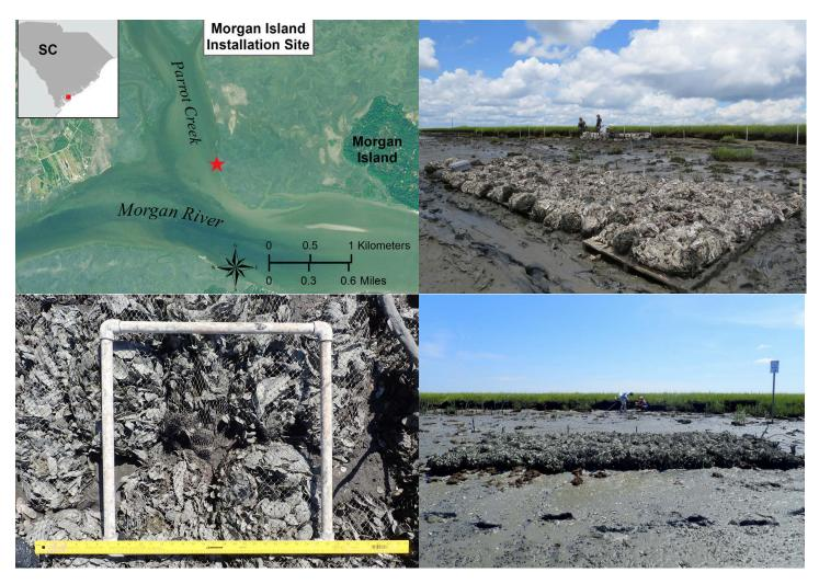
**Figure 3.6.** Aerial view of the living shoreline research site on Morgan Island (upper left). Shell bag constructed on wooden pallets in July 2016 (upper right). Percent oyster coverage (lower left) and shell bag reef (lower right) in August 2018.
