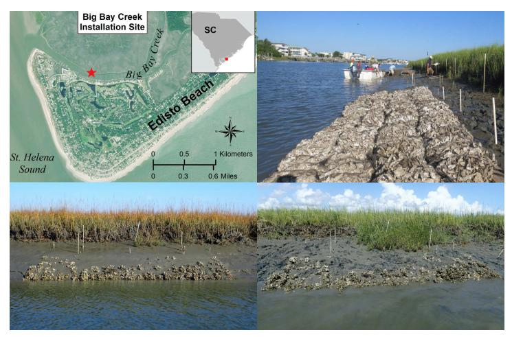
**Figure 3.4.** Aerial view of the living shoreline research site on Big Bay Creek (upper left). Shell bag reef constructed on wooden pallets in July 2016 (upper right). Oyster growth and sediment accumulation on reef at Big Bay Creek in November 2017 (one year post-install; lower left) and in September 2018 (two years post-install; lower right). Note marsh grass expansion (lower right).
