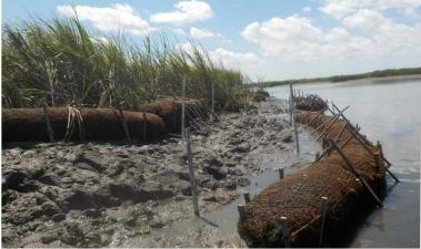
**Figure 3.15.** Coir rope laced through stakes and tied to secure log in place (upper left). Bagged oyster shell was used in front of some coir logs to prevent undercutting of the log but was later discontinued (upper right). Double-row coir log at Orangegrove Creek, with alternate A-frame staking, installed in August 2017 (lower left).
