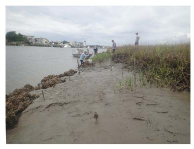
**Figure 3.10**. Almost 3 years after installation of the MWR at Big Bay Creek, oyster cover and growth continue to increase, and marsh expansion was starting to occur. Photo taken in May 2019.
