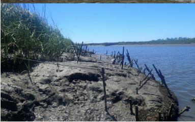
**Figure 3.20.** A double-row coir log treatment at Orangegrove Creek in August 2017 (top). The same coir log treatment in May 2018, with smooth cordgrass freshly planted in the sediment trapped between the logs (middle); full view (bottom left) in April 2019.
