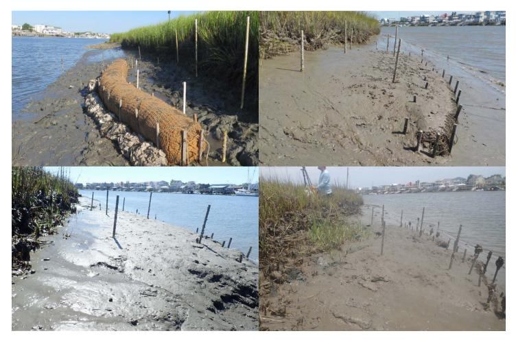
**Figure 3.16.** A single-row coir log treatment at Big Bay Creek (Figure 3.4) in July 2016 (upper left), October 2017 (upper right), September 2018 (lower left), and May 2019 (lower right).
