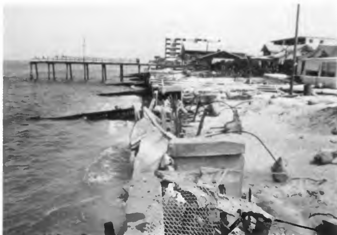
a) September 9, 1985, within One Week after Hurricane Elena.
