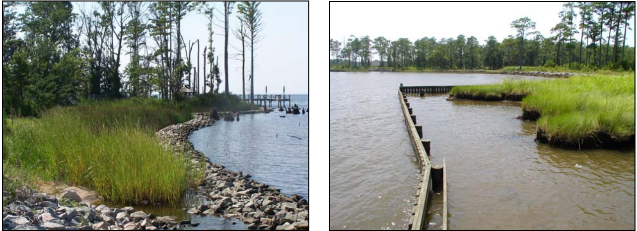
Figure 5-6: View of a rubble mound (rock) sill (left) and a timber sheet pile sill (right).
