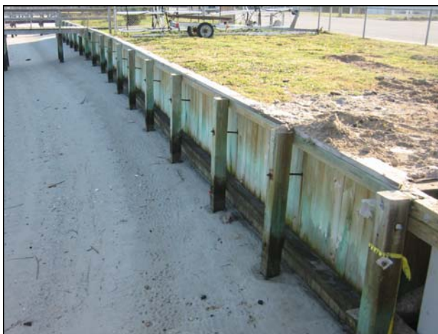
Figure 5-17: Typical CCA treated timber bulkhead (left) and stone seawall (left).
