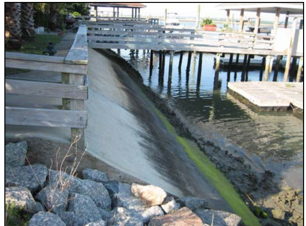
Figure 5-14: Sloped structures constructed from rock (left) and watertight cast concrete (right).
