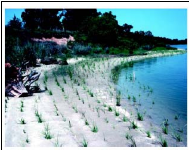
Figure 5-1: Vegetation Control in the form of marsh planting (left) and its growth after 1 year (right). (Barnard and Hardaway)
