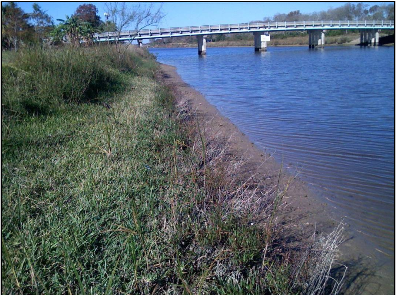
Figure 16. BEFORE: Scarborough shoreline before grading and planting
