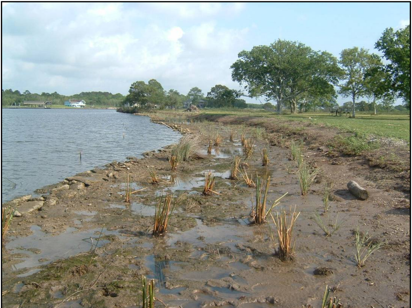
Figure 11. DURING: Planting in constructed fill area behind rock breakwater at Asher site
