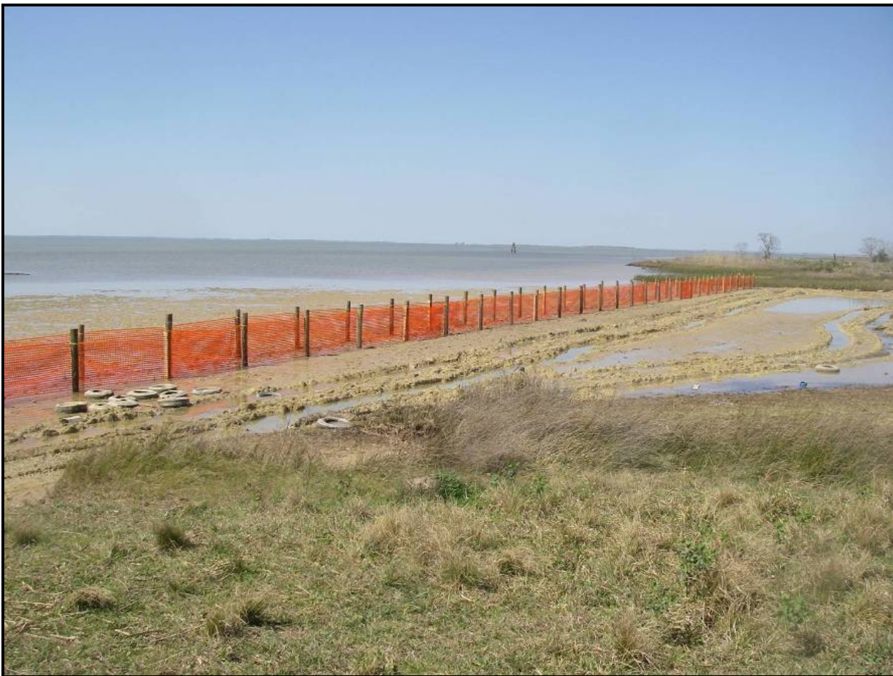
Figure 18. Double-row erosion control fencing
