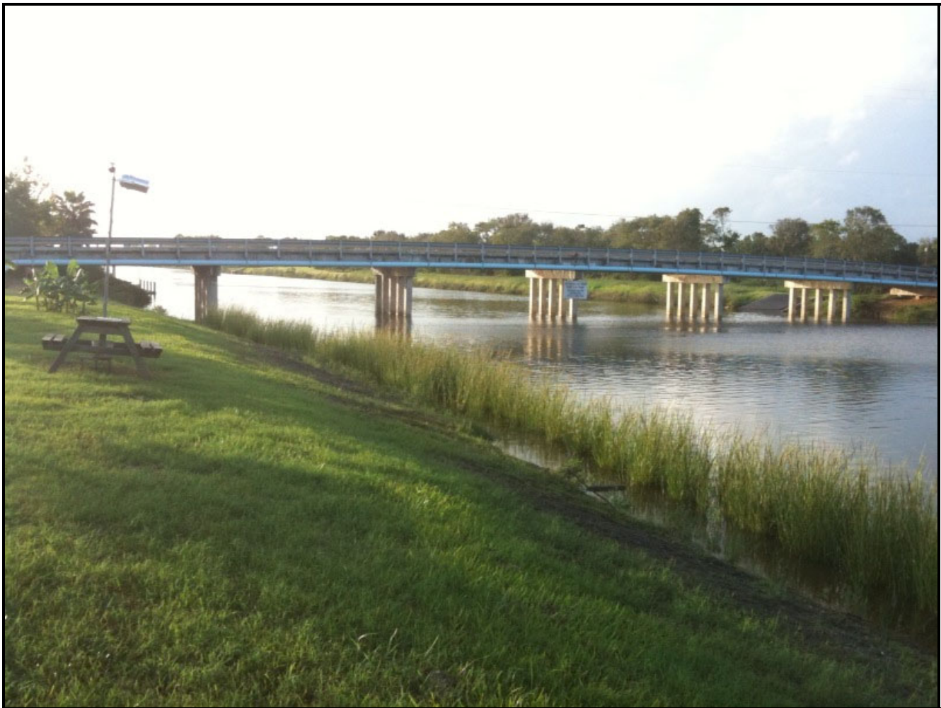
Figure 17. AFTER: Scarborough shoreline six months after planting Photo: Tom Scarborough
