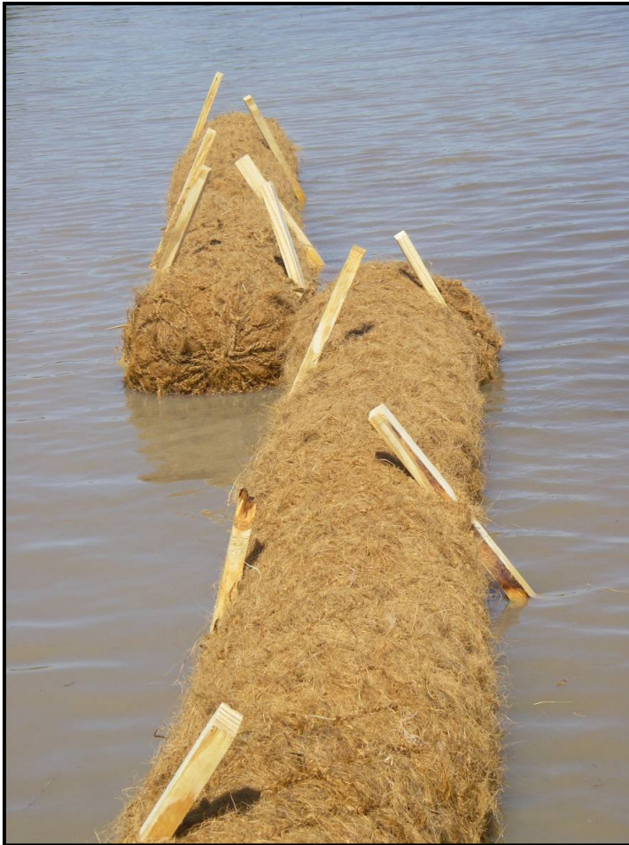
Figure 20. Staked coir logs
