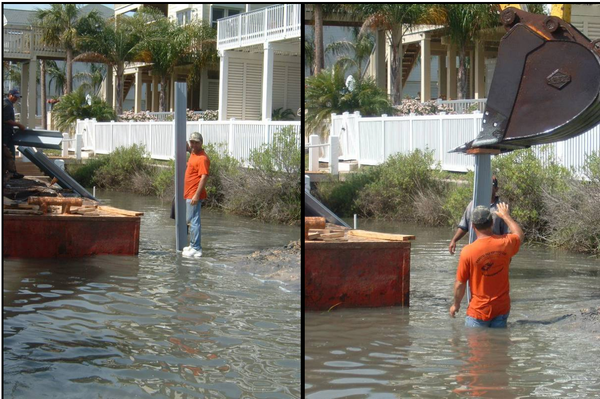
Figure 14. DURING: Vinyl sheetpile installation
