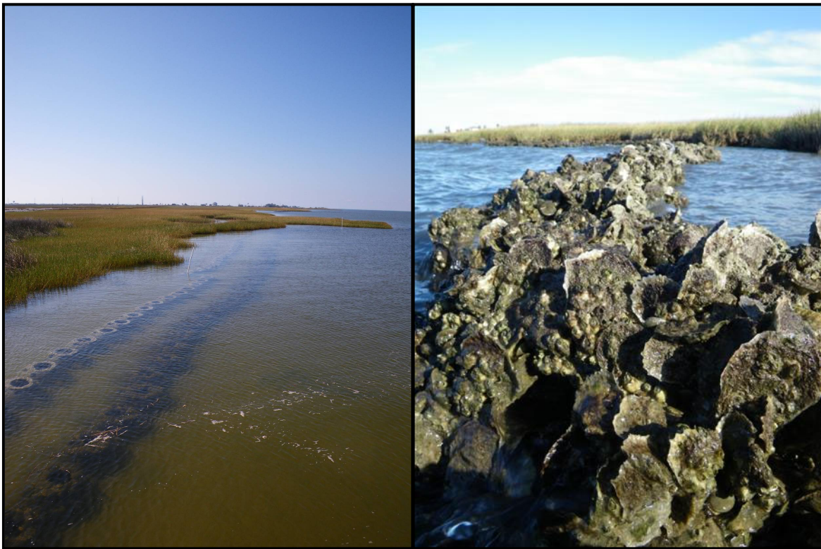
Figure 13. Reef domes installed at Sweetwater (left), encrusted with oysters (right)
