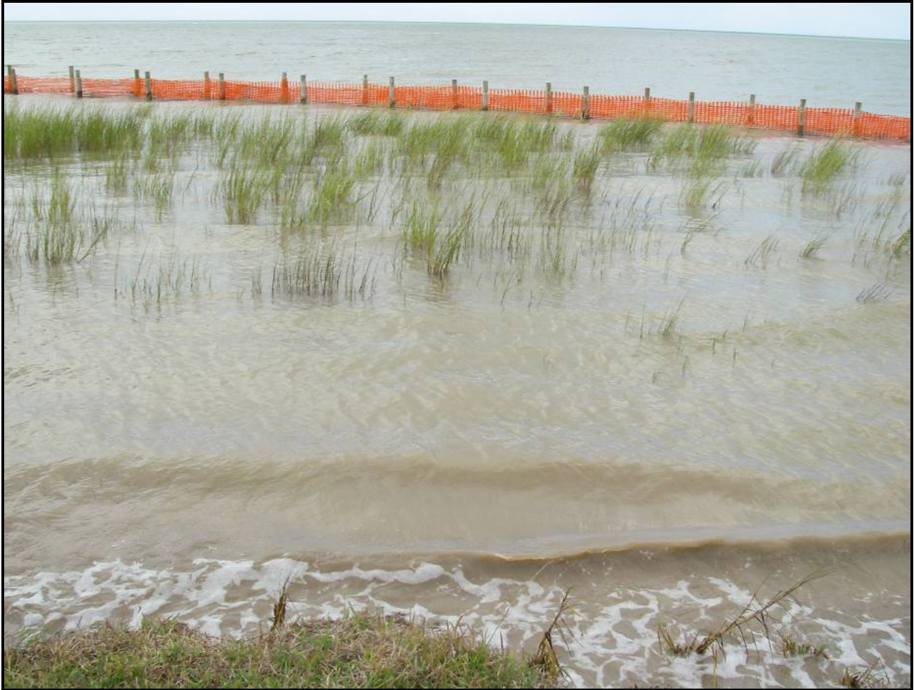
Figure 19. Planting behind erosion control fence
