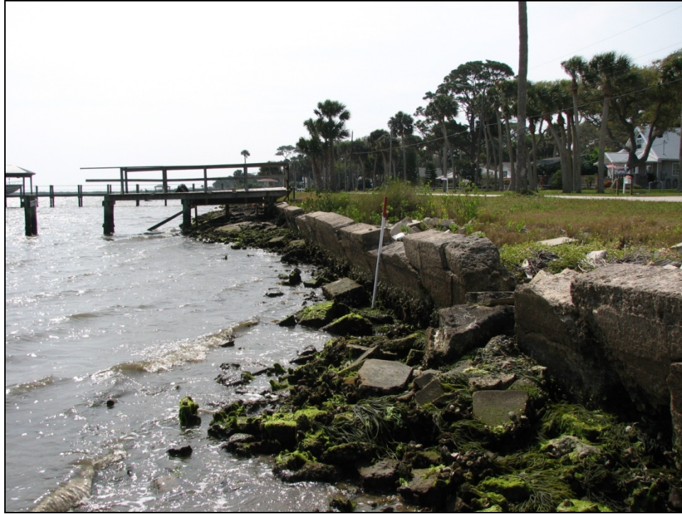
Figure 13. Transect 57 South View – Bulkhead is deteriorating. Inappropriate riprap and no salt marsh vegetation or oyster habitat.
