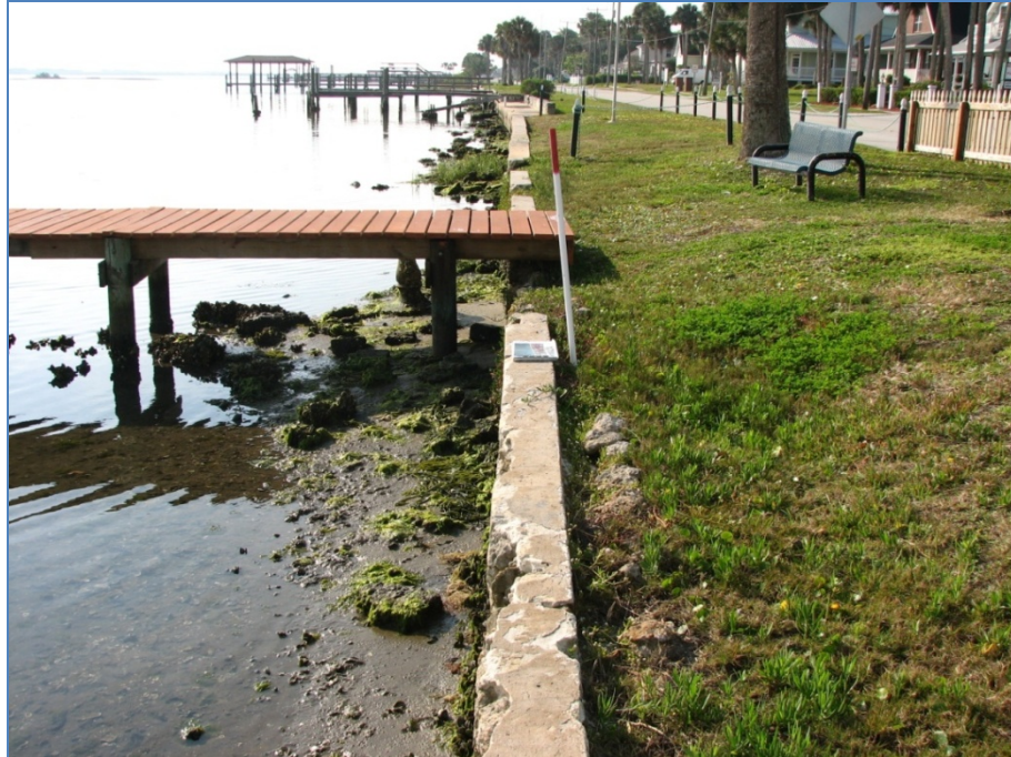
Figure 11. Transect 32 South View. The bulkhead appears stable, though there is some erosion apparent behind the bulkhead. There is no salt marsh vegetation or oyster habitat in the vicinity.
