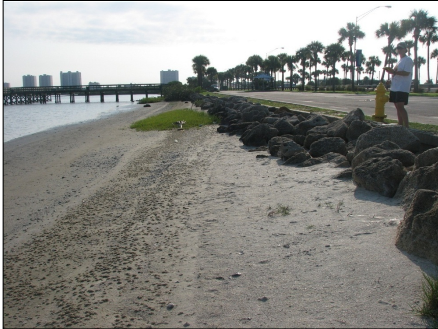
Figure 17. Transect 172 East - Bulkhead with riprap. There is a small patch of salt marsh vegetation.
