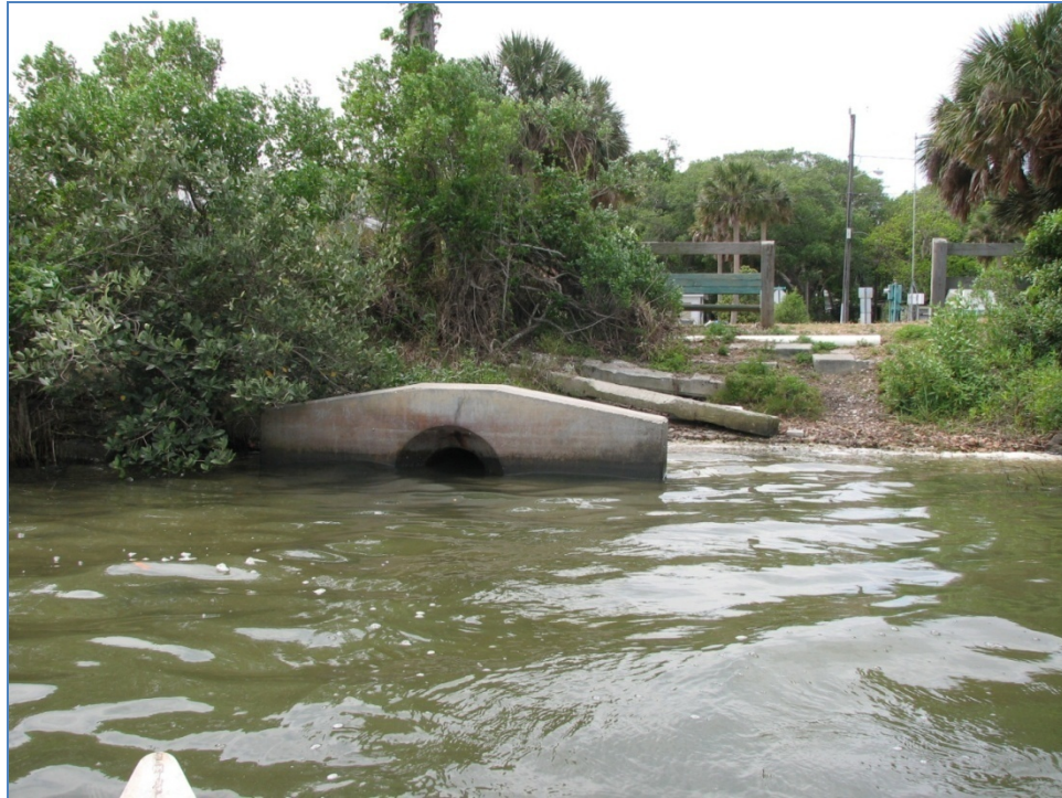
Figure 15. Transect 153 looking west. The area contains a large stormwater outfall, and eroded shoreline with large concrete debris
