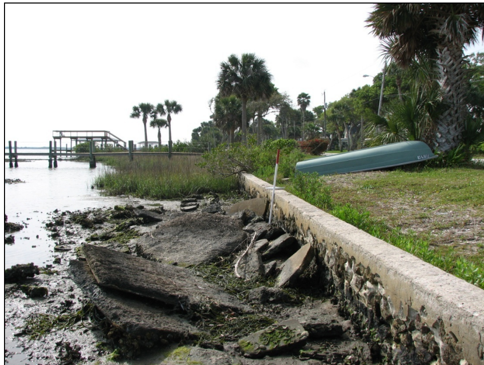
Figure 12. Transect 46 South. - Inappropriate riprap and no salt marsh vegetation or oyster habitat.
