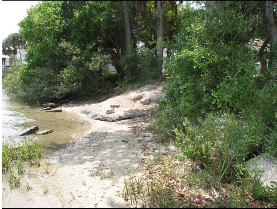
Figure 16. Transect 161 South - Severely eroded shoreline with scattered riprap. Some Spartina present.
