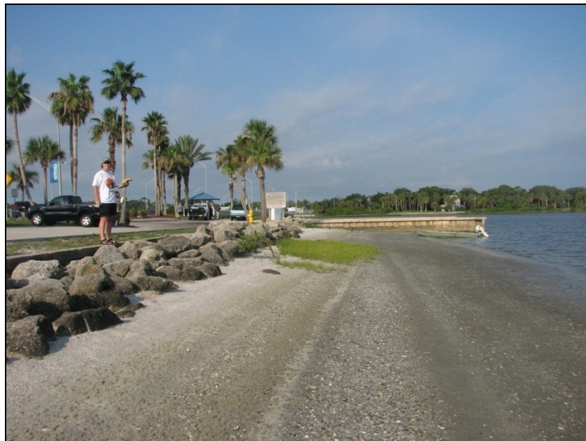
Figure 18. Transect 173 West View- Bulkhead with riprap. No salt marsh vegetation or oyster habitat.
