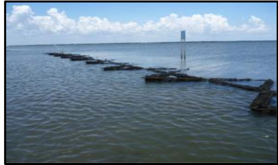
Figure 16. ReefBlk TM structures installed at Coffee Island, AL. Steve Jones.
