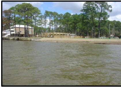
Figure 9. Revetment. Mobile Bay, AL. Steve Jones.
