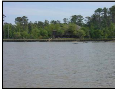
Figure 10. Wooden Bulkhead. Mobile Bay, AL. Steve Jones.
