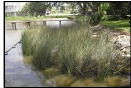
Figure 13. Wooden Sill. Mobile, AL. Scott Douglass.
