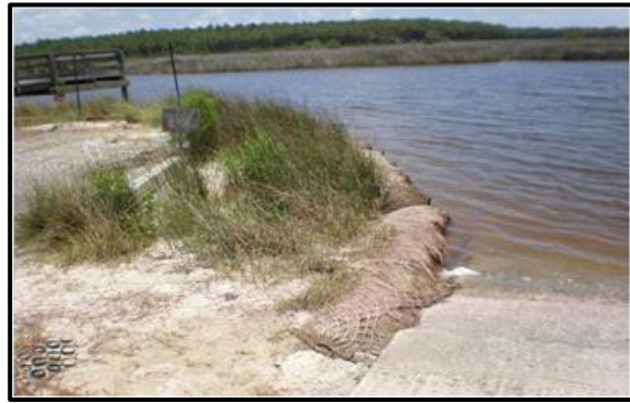
Figure 5. Coir fiber with vegetative planting. Moss Point, MS. Chris Boyd.
