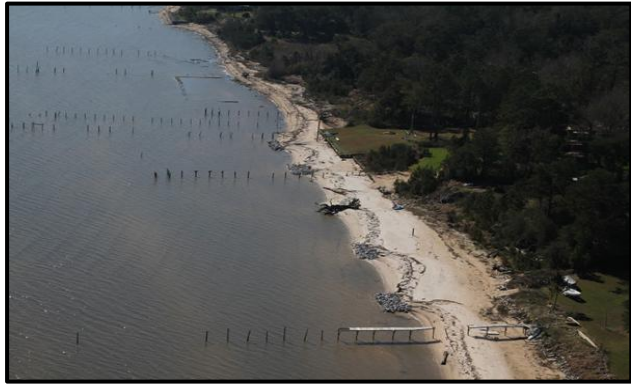
Figure 18. Breakwaters Installed to create protected headlands. Mon Louis Island, AL. Tom Herder.
