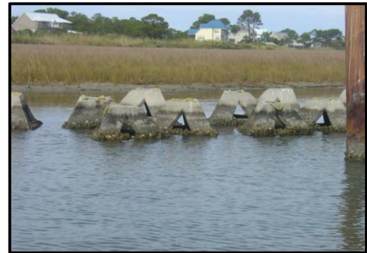
Figure 14. Wave Attenuation Devices, Dauphin Island, AL. Steve Jones.
