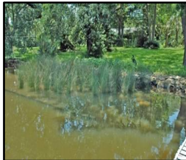
Figure 7, Wooden breakwater with vegetative planting. Mobile, AL. Scott Douglass.
