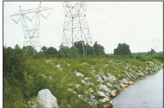
Figure 8: Typical Joint Planted Revetment
